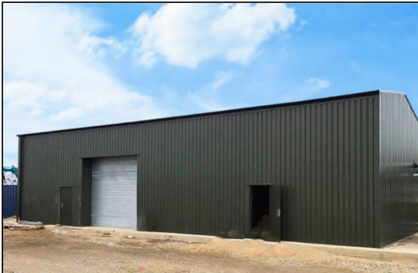
Plate 3.11: Example of a Collector Compound
